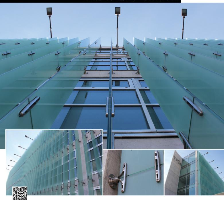
GLASSCON developed, fabricated and installed an innovative solar shading system consisting of vertical architectural SOLAR GLASS LOUVERS as a complete building envelope. After comprehensive shading study, the selected system allows undisturbed view from the interior of the building, whilst providing efficient
