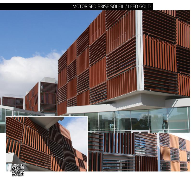
GLASSCON was involved in the rehabilitation works of an office building complex, including the design, engineering, fabrication and installation of an architectural second skin which contributed the most to building's LEED Gold certification. The kinetic solar shading system combines solar gain
