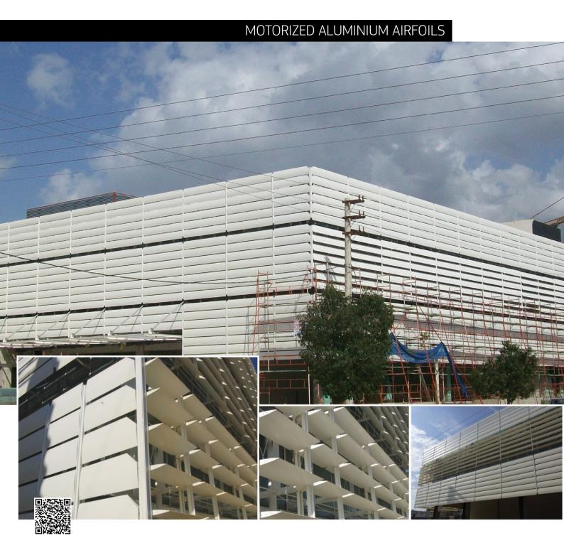
GLASSCON designed, engineered and constructed a fully motorized external shading system with ALUMINIUM AIRFOILS for a telecommunications office building. The selected material has an aero blade shape and is certified for its rigidity and durability. According to the solar shading study results, the whole façade had to be totally
