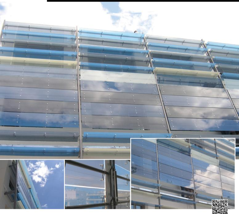
GLASSCON designed, fabricated and installed an innovative second skin shading system for an eye clinic with MOVABLE GLASS LOUVERS operating fully automated. The glass louvers carry silk printing to create the desired transparency and provide efficient shading. Glass used is tempered
