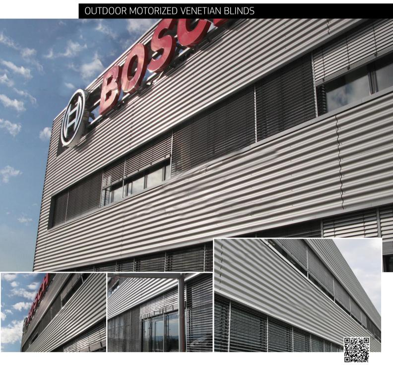
GLASSCON successfully executed the complete façade works for a Bosch office building including external motorized venetian blinds and aluminium corrugated sheet cladding. This shading system provides easy and high efficient shading options through rotation and vertical sliding to any stack position, during all periods of
